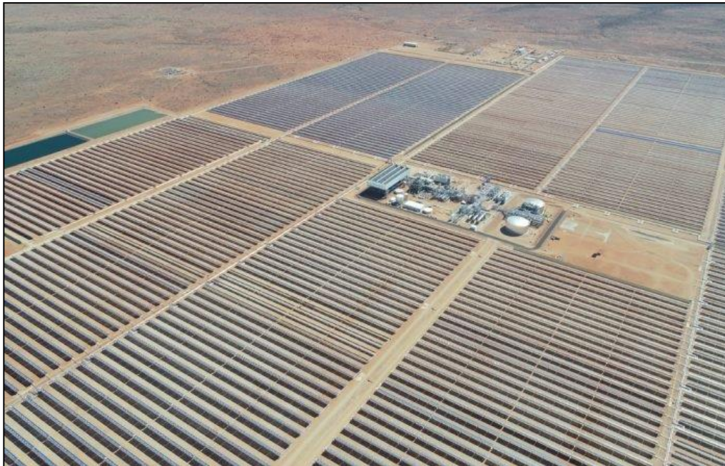
Figure 3: Ilanga CSP solar energy power plant, Northern Cape
